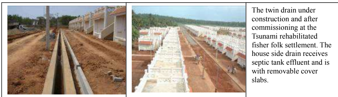
Figure 3.11 Twin drain system
