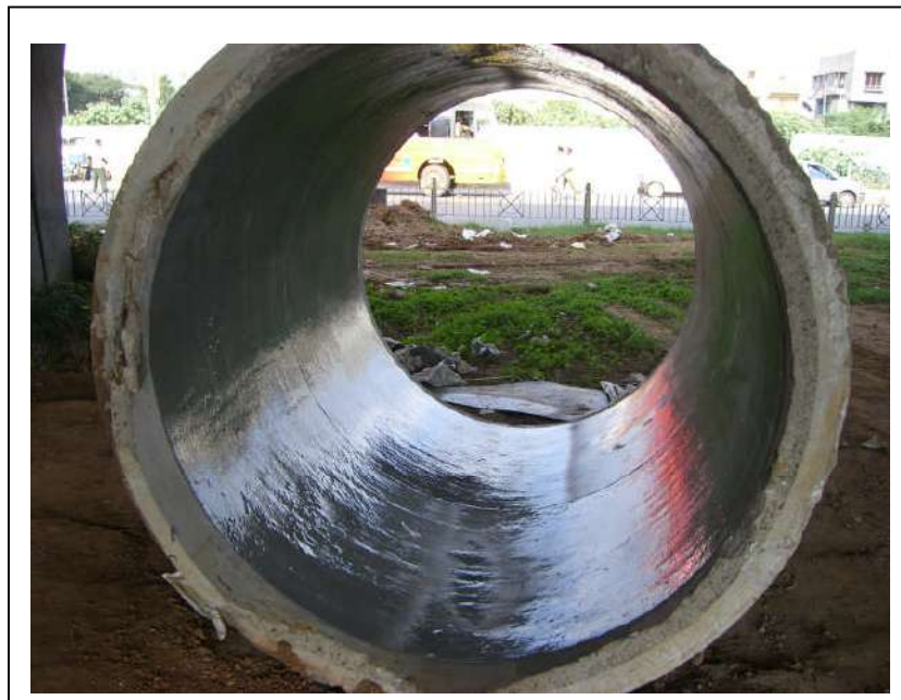
Figure 3.58 RCC Sewer pipe with protective coating
