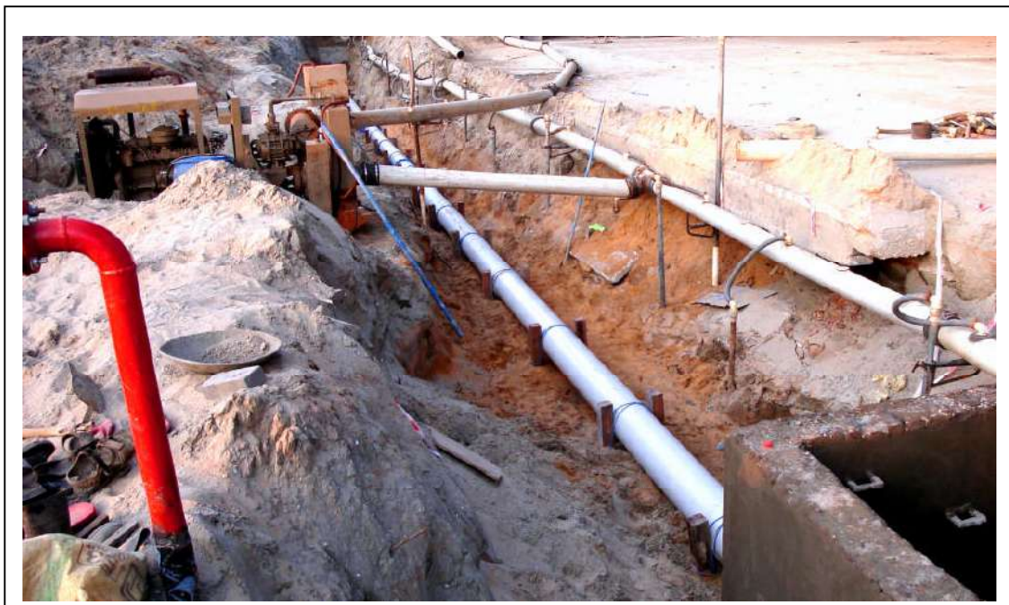
Figure 3.45 Typical arrangements for laying sewers in high subsoil locations using dewatering pump sets, tube wells and Venteak piles with cross brace and nylon rope wrapping around the sewers securing it to the venteak piles and brace
