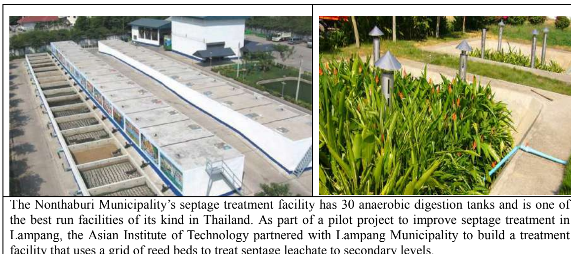
Figure 9.22 A photo view of septage treatment process at Nonthaburi in Thailand
