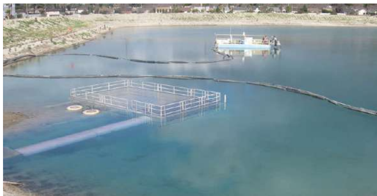
Figure 7.12 Purified water from the GWRS is piped to OCWD's percolation ponds in Anaheim, California
