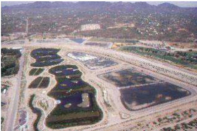
Sweetwater SAT treatment plant, Tucson, AZ
