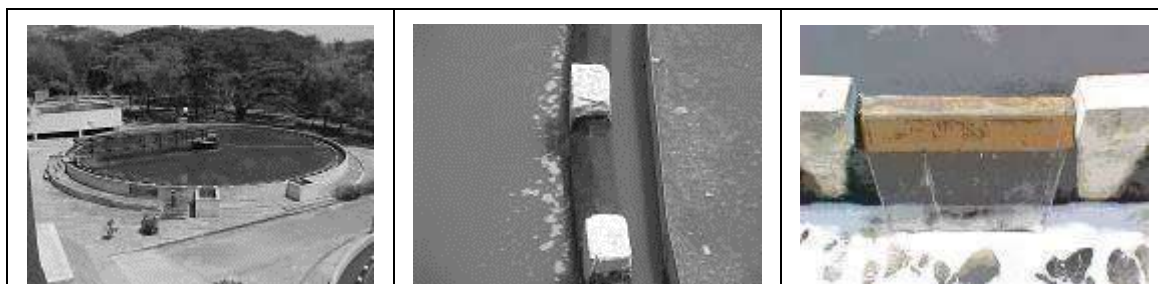
Figure 5.29 Left and middle are the primary clarifiers. At right is the secondary clarifier. The free fall permits additional entrainment aeration of the secondary treated sewage.
