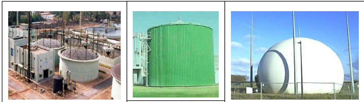
Figure 6.12 Some views of gas holders.
