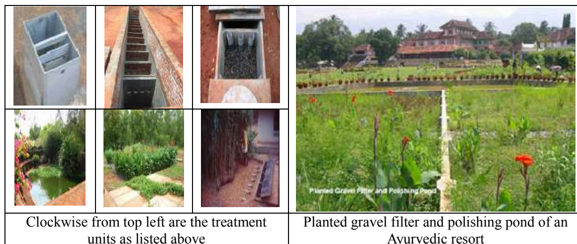
Figure 8.14 Typical DEWATS treatment plant components
