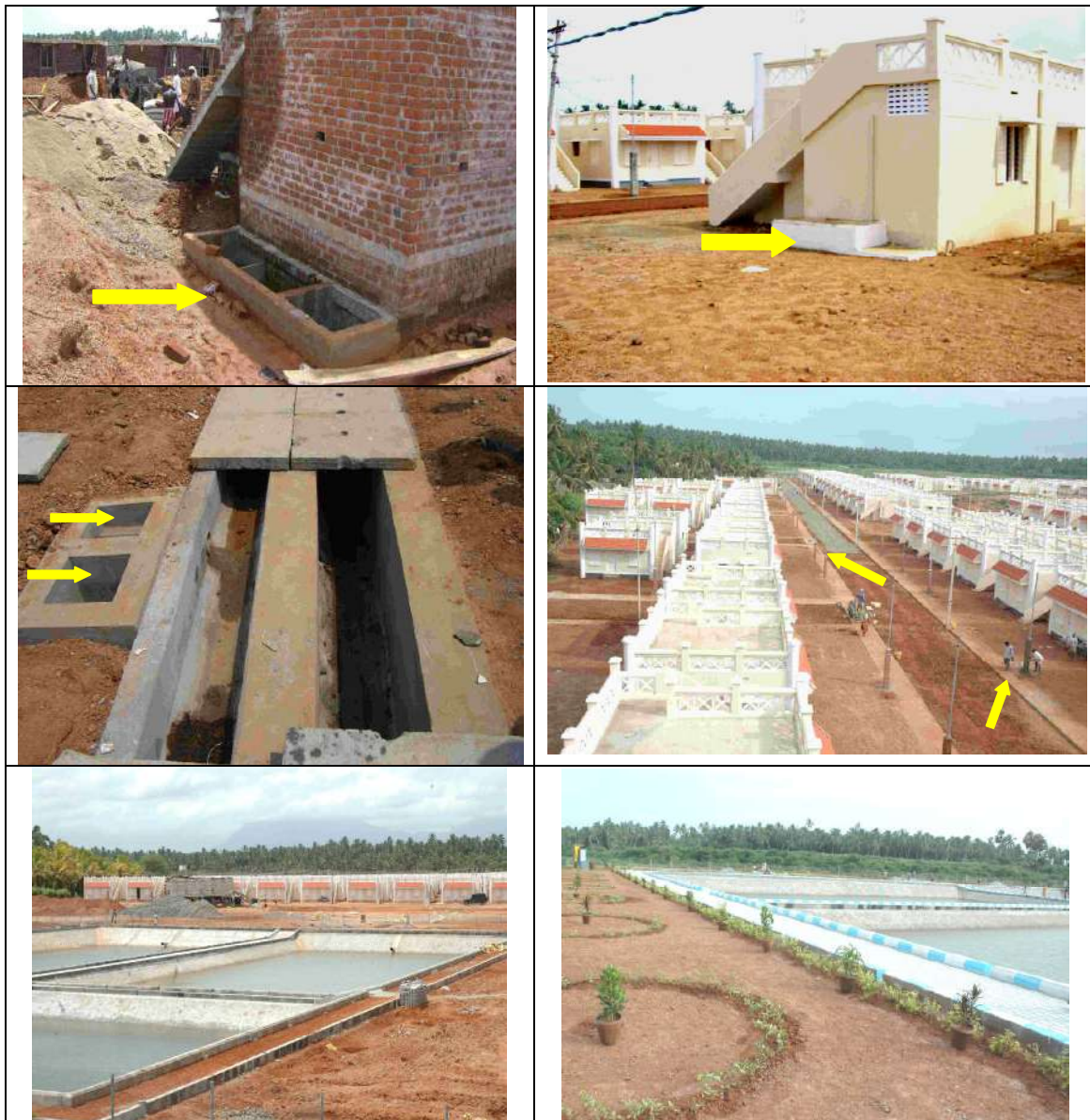
Figure 8.8 Schematic of the twin drain decentralized sewerage
